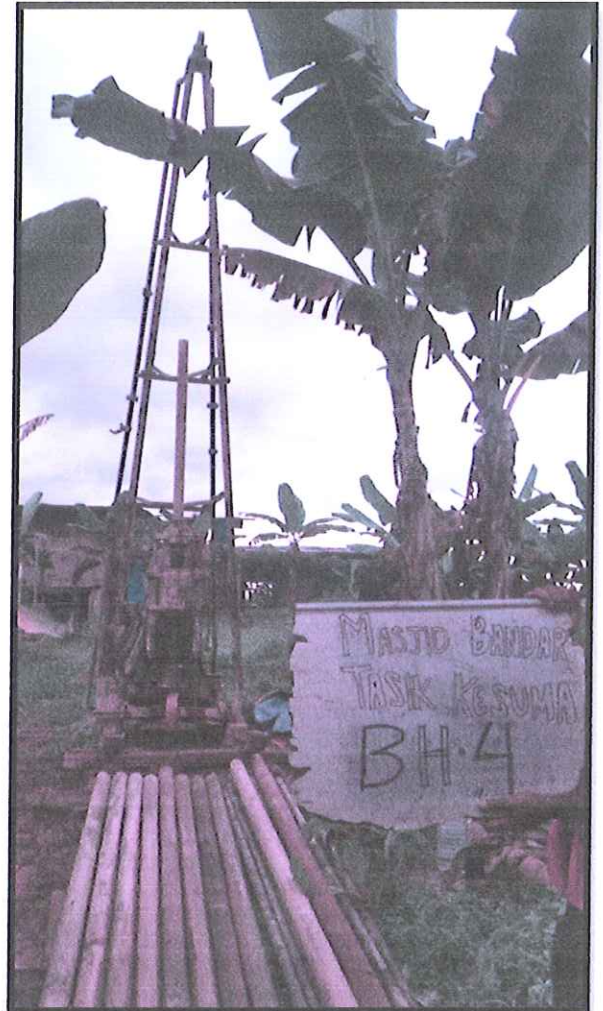
DRILLING OPERATION BH 4 TERMINATION DEPTH: 30.25m
