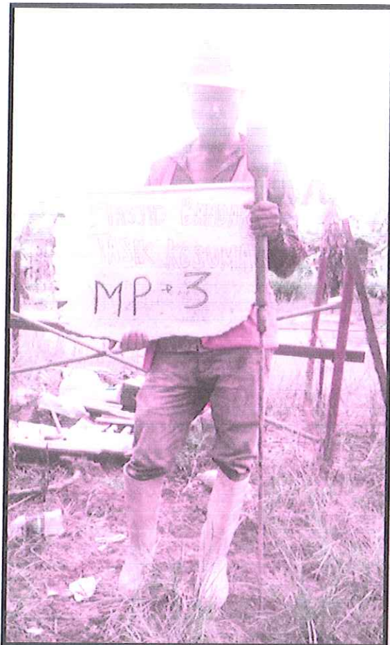
Carry out Mackintosh Probe at MP 3
