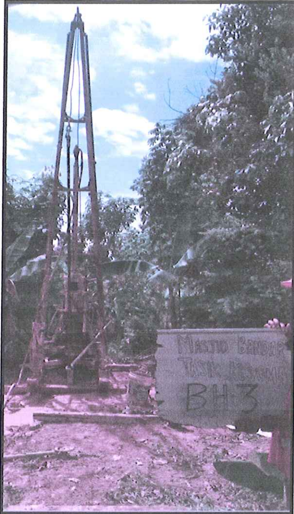
DRILLING OPERATION BH 3 TERMINATION DEPTH: 27.18m
